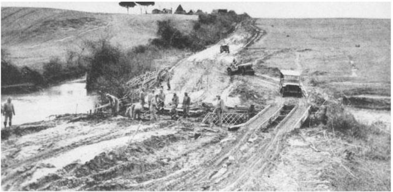
ENGINEERS BRIDGE A STREAM on a road from Nettuno to the front. Frequent rains and enemy shell-fire damage made this a difficult task, but the roads had to be kept open to move armor against the Germans
